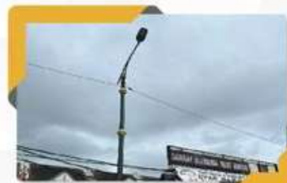
Kerja-Kerja Pemasangan 8 Unit Smart Street Lighting System Di Dataran Alamanda Pusat Bandar, Parit Buntar (Negeri - P07)
